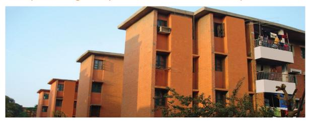
A brick stone elevation of Group Housing Complex was built for Indian Agriculture Research Institute Pusa. An extensive area spread over approximately 1,18,790 sq. ft. stands tall as a fine example of unparralleled construction standards in affordable housing schemes. The RCC framed, G+3 storeyed structure is built on a raft foundation including allied development works, completed within a span of 2 years. This project of NRI received much acclaim due to timely deliverance and quality.
